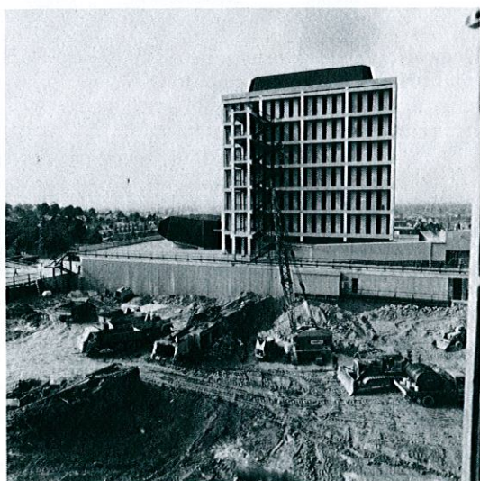
Stage 1 Building in progress.
